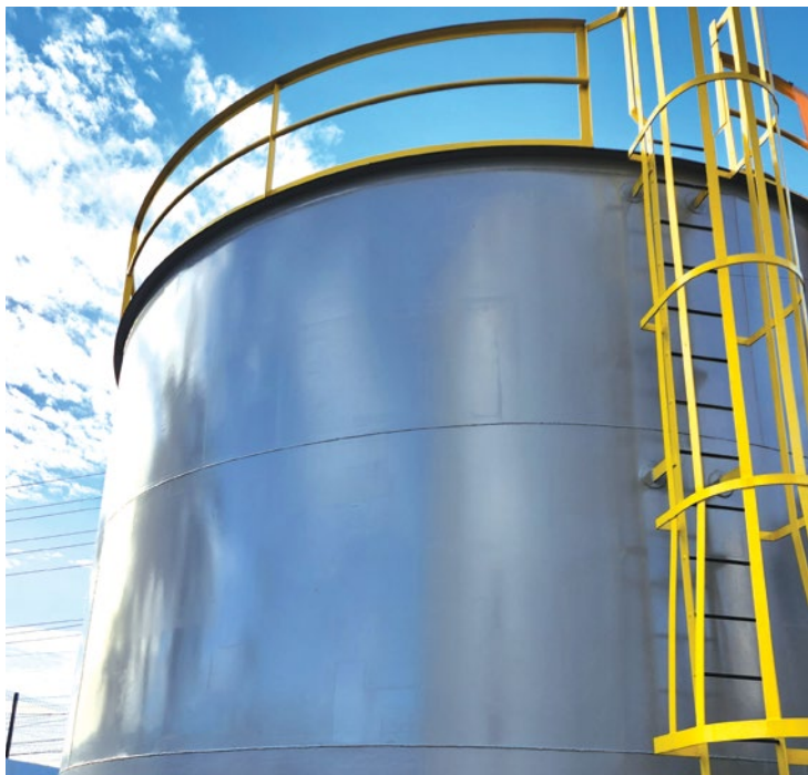
Repaired Fire Fighting Water Tank
