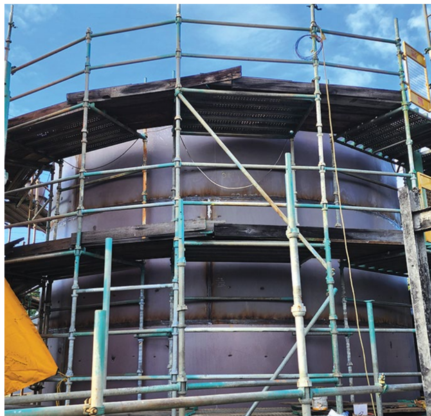
Water storage tank being repaired
