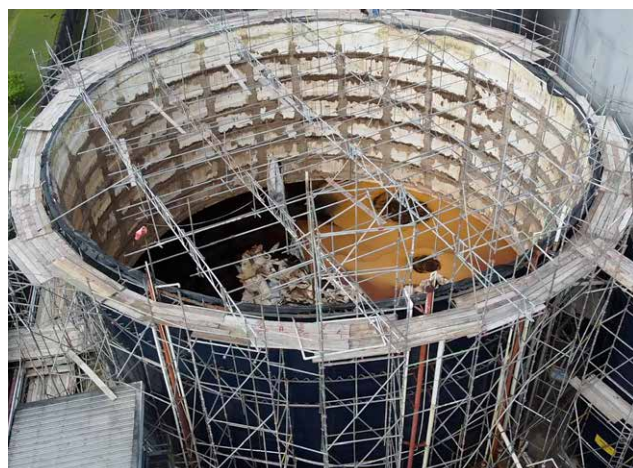
Removal of the Roof on the Anaerobic Digester in preparation for emptying
